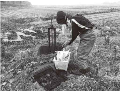
St.C: Culvert pit
