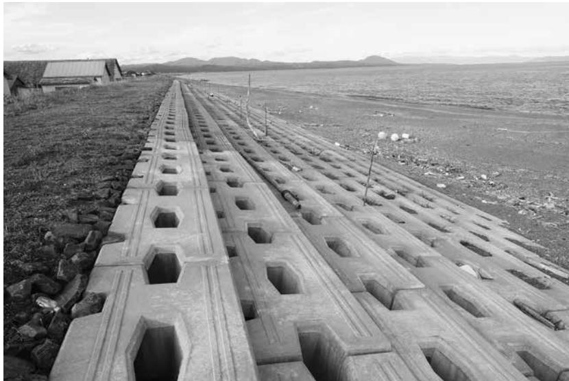
Photo 3. Stepped armor blocks and their holes at site B
